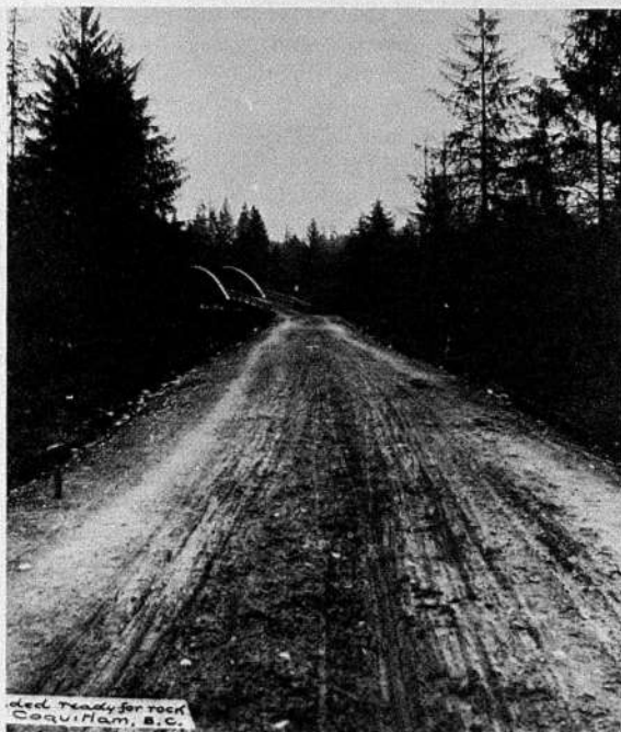
Graded, ready for rock, Coquitlam, B.C.
