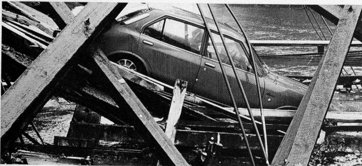
'Red Bridge Collapse', October 26, 1982. A total of five cars were left stranded when an out-of-control vehicle hit one of the main supports of this Pitt River Road crossing of the Coquitlam River. Photograph Colin Morris.
