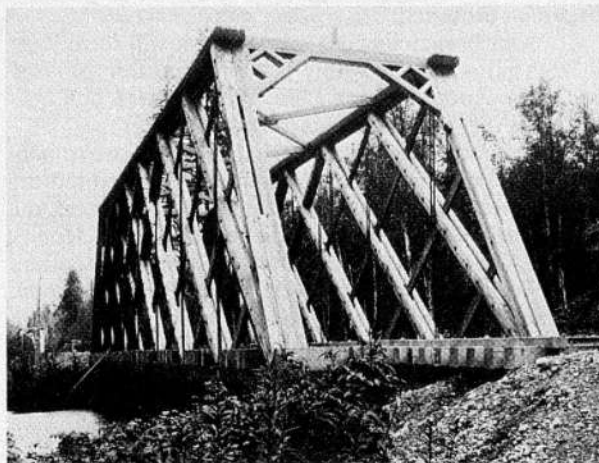
Pre-fabricated wooden rail bridge near Westminster Junction. From the Onderdonk photographic album, Courtesy B.C. Provincial Archives.
